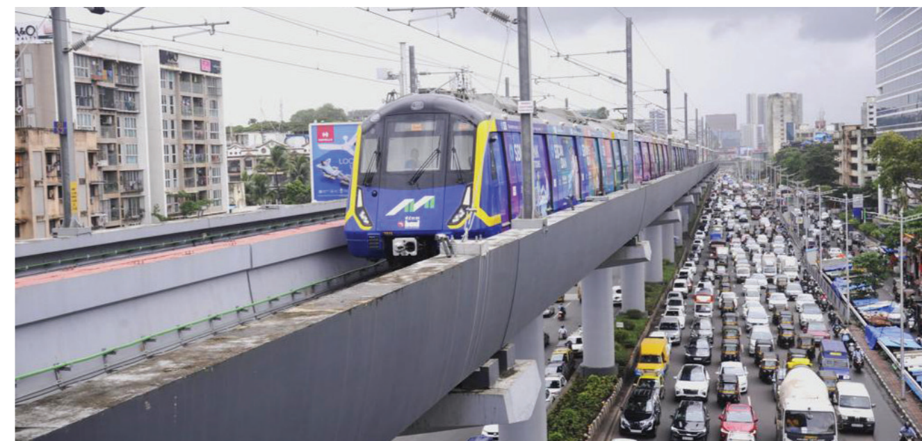
REC funded Mumbai Metro Project
