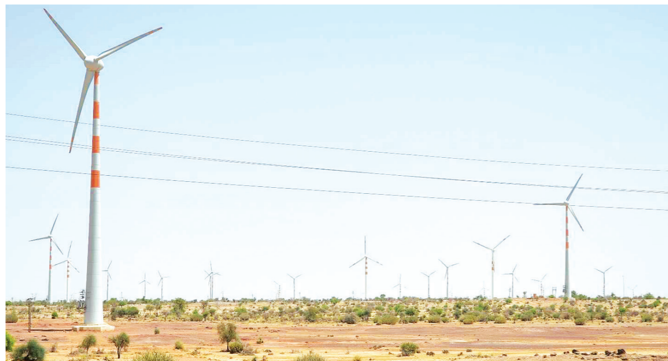
REC funded 100 MW Wind Energy Project in Rajasthan
