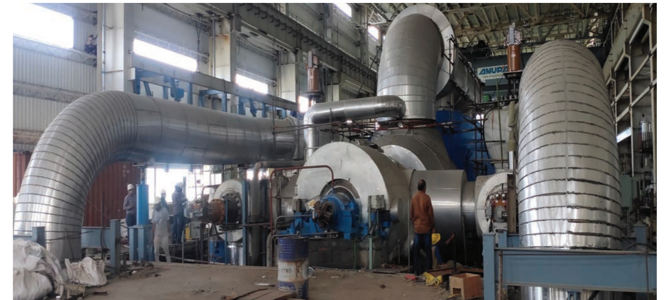
REC financed 800 MW Dr. Narla Tata Rao Thermal Power Station Stage-V Project at Vijayawada
