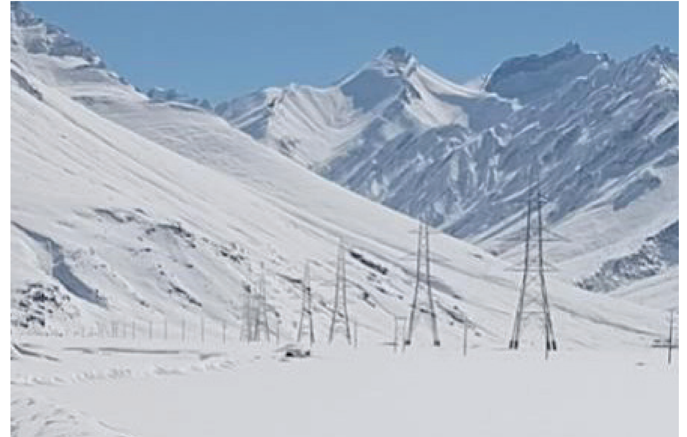
220kV Single Circuit Transmission Line from Drass to Padum on Double Circuit Tower at Kargil, Ladakh being implemented by RECPDCL
